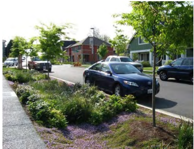
Bioswales located in public rights-of-way are particularly affective in reducing the stormwater flow and improving quality for stormwater that falls on roadways.
