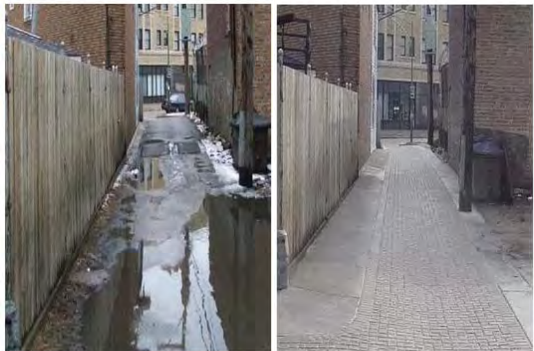
Alley with flooding issues prior to instillation of pervious pavers (left) and after (right). Photos: Courtesy of CMAP
