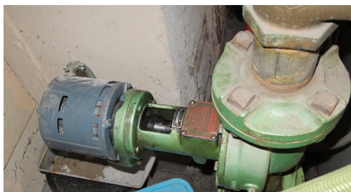
Figure 16. Primary circulator at Building B
