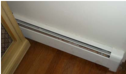
Figure 6. Baseboard radiator (left); radiant flooring (right)
