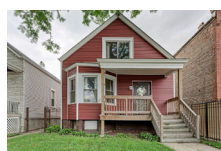
Single family, Pre-1942 Frame construction Qty: 1,769
