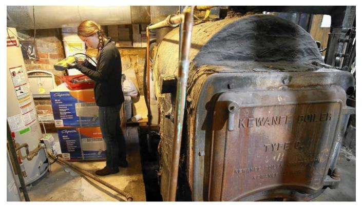
During a recent energy audit, Tessa Maurer of nonprofit Elevate Energy checks an old boiler in a North Side apartment building. She recommended replacing the boiler. (Alex Garcia, Chicago Tribune)
